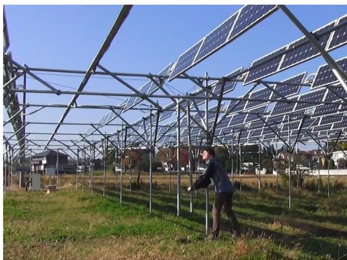
**Figure 1.2 Movable solar photovoltaic panels in AV system (Source: <https://solar-sharing-japan.blogspot.com/2014/>).**
