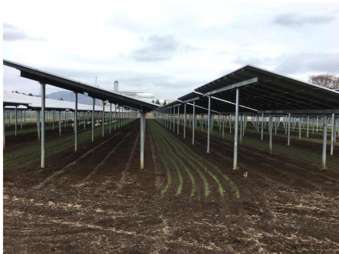
**Figure 1.1 Fixed solar photovoltaic panels in AV system.**
